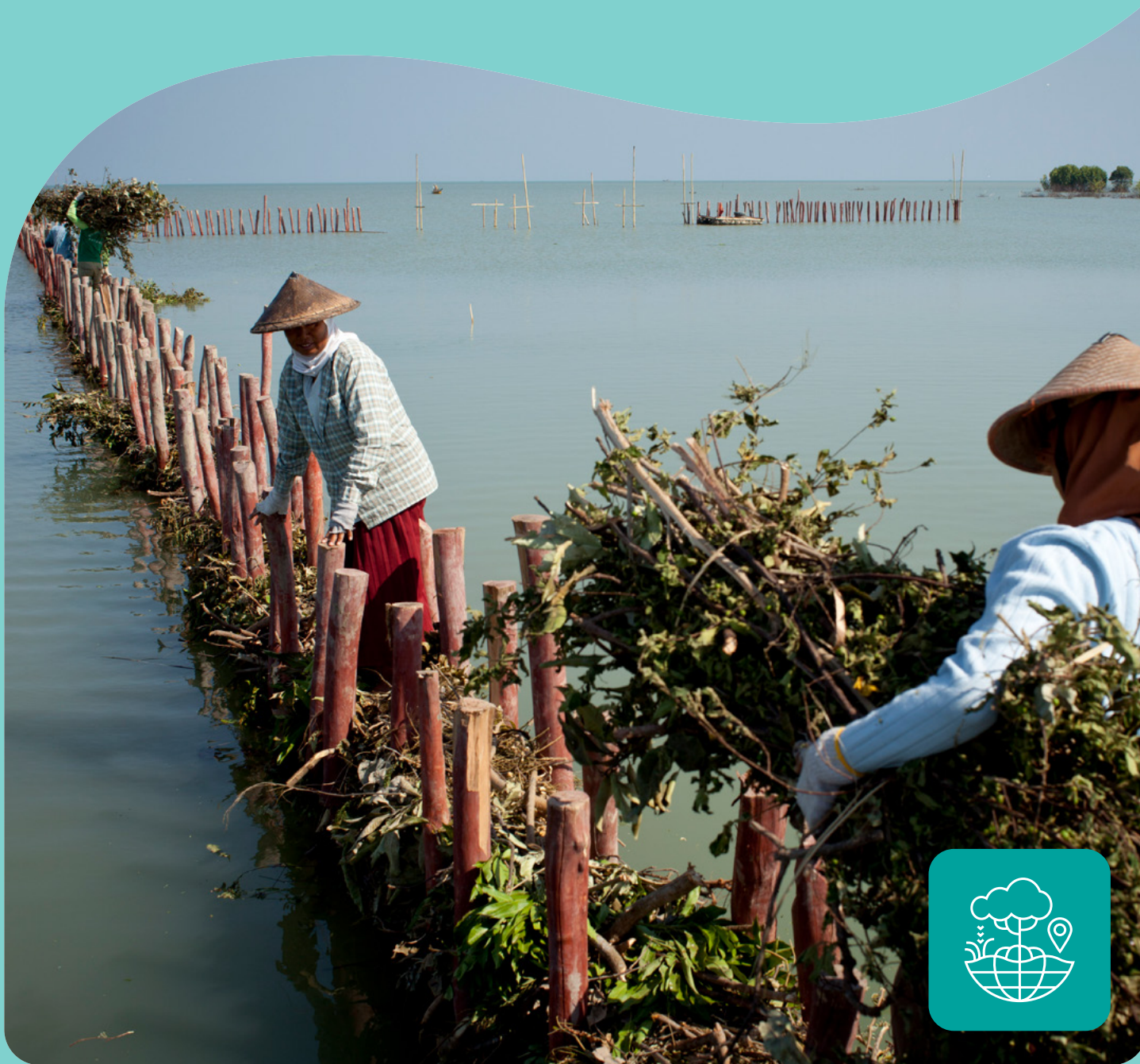
Community groups constructing permeable structures to trap sediment in Demak, Indonesia © Nanang Sujana
